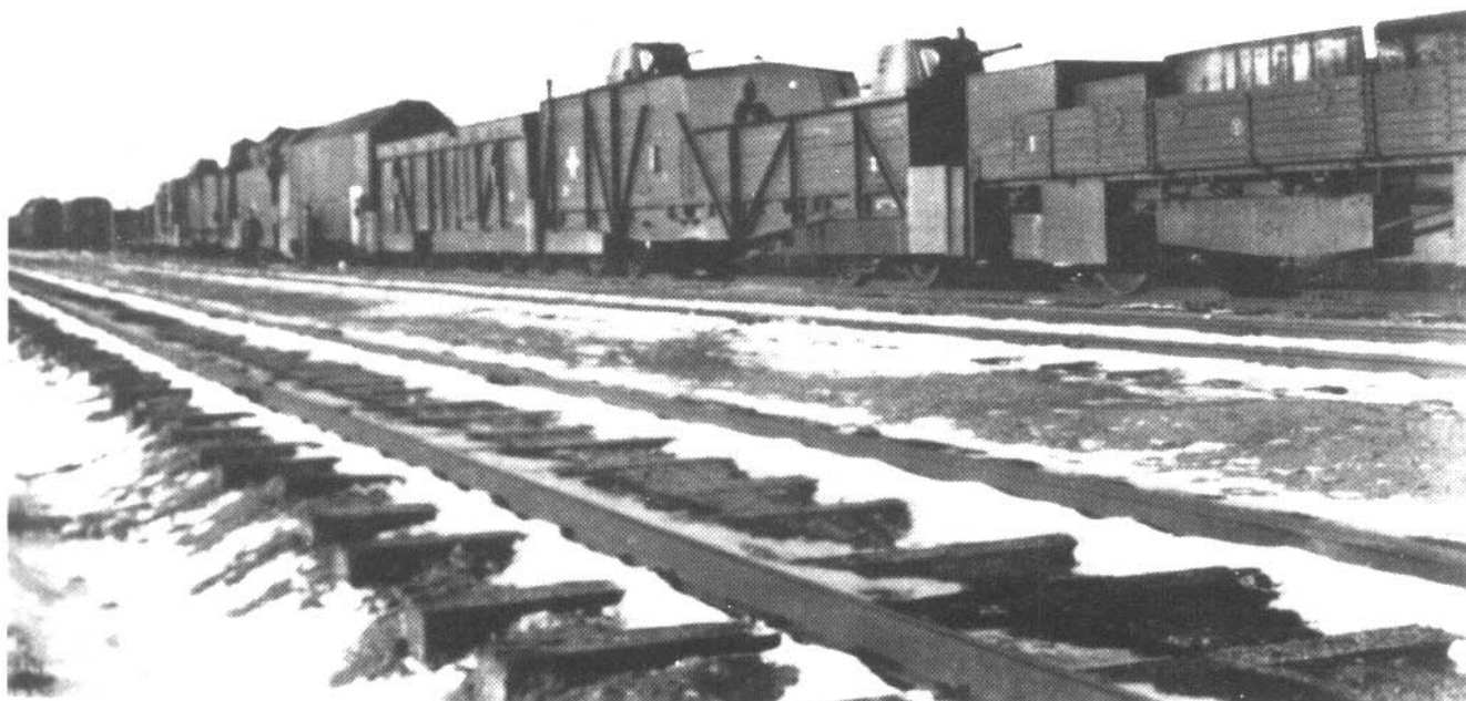
In the spring of 1942 a railway protection train (captured Russian freight cars, armored inside) was upgraded to PZ 51. Kept from its Soviet state was the mounting of tank turrets (here Russian BT-7) as gun mounts.
