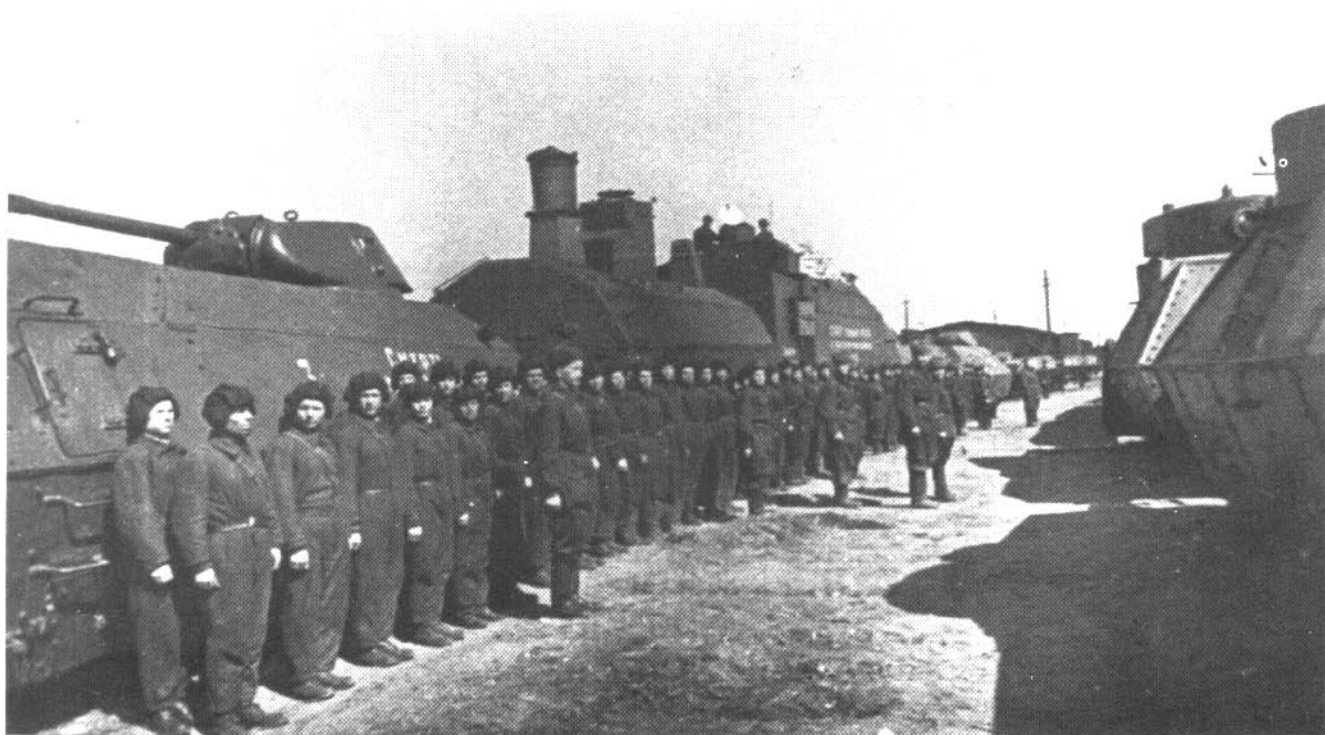
Two Soviet armored train designs of 1942: At right an OB-3 with four two-axle cars, each with one gun turret (7.62 cm 02/30 gun); at left the further development of NKPS-42 (two four-axle cars with two turrets each) with T-24 tank turrets. This armament (see also back cover) became the Russian standard in 1943. (PM)
